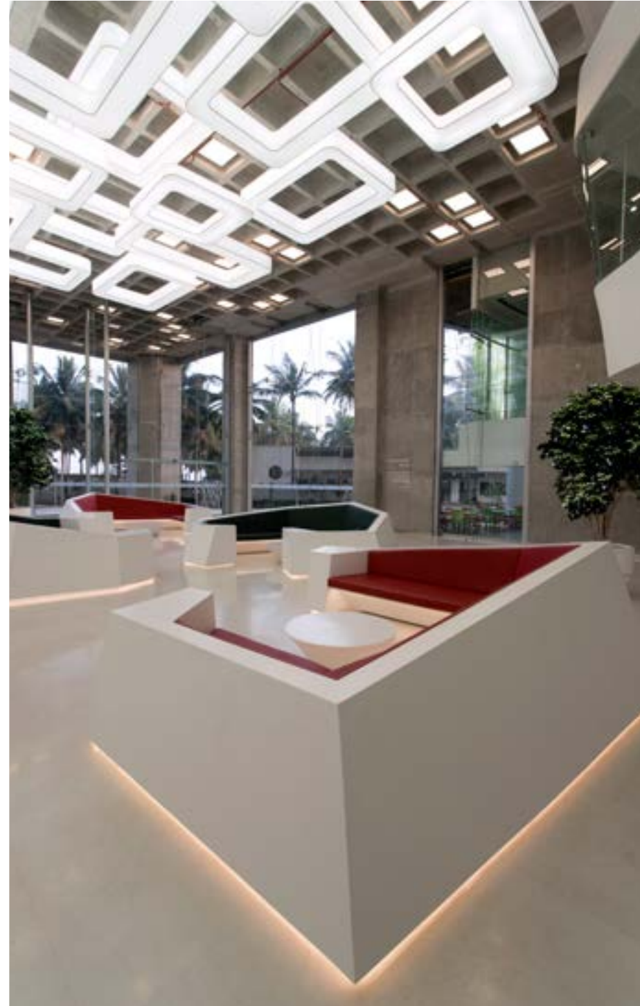
The waffle slab system is left exposed to contrast against the stark light fixtures and white interiors
